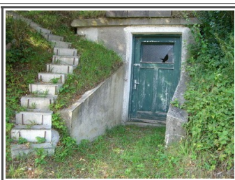
Die alte Wasserreserve in Arlesried.
